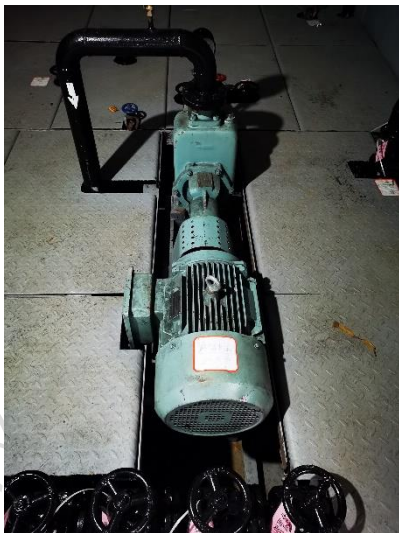
码头生产废水污水水泵
